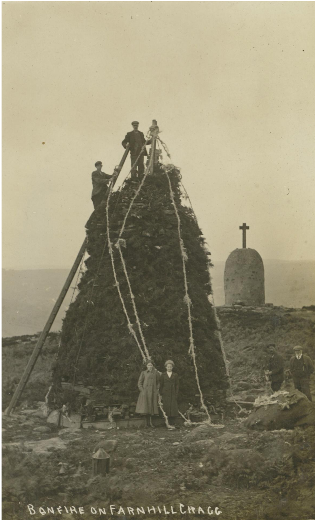
Figure 2a: The bonfire being built on Farnhill Moor
